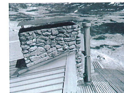
PHOTO: 8 - 10 = ROOF DETAILS
